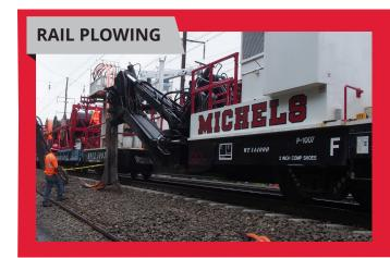
Rail plowing is a quick, effective way to install cables and conduit along railway rights-of-way. Our proprietary rail-mounted plows facilitate the installation or upgrade of fiber optic cable and signal wire.
